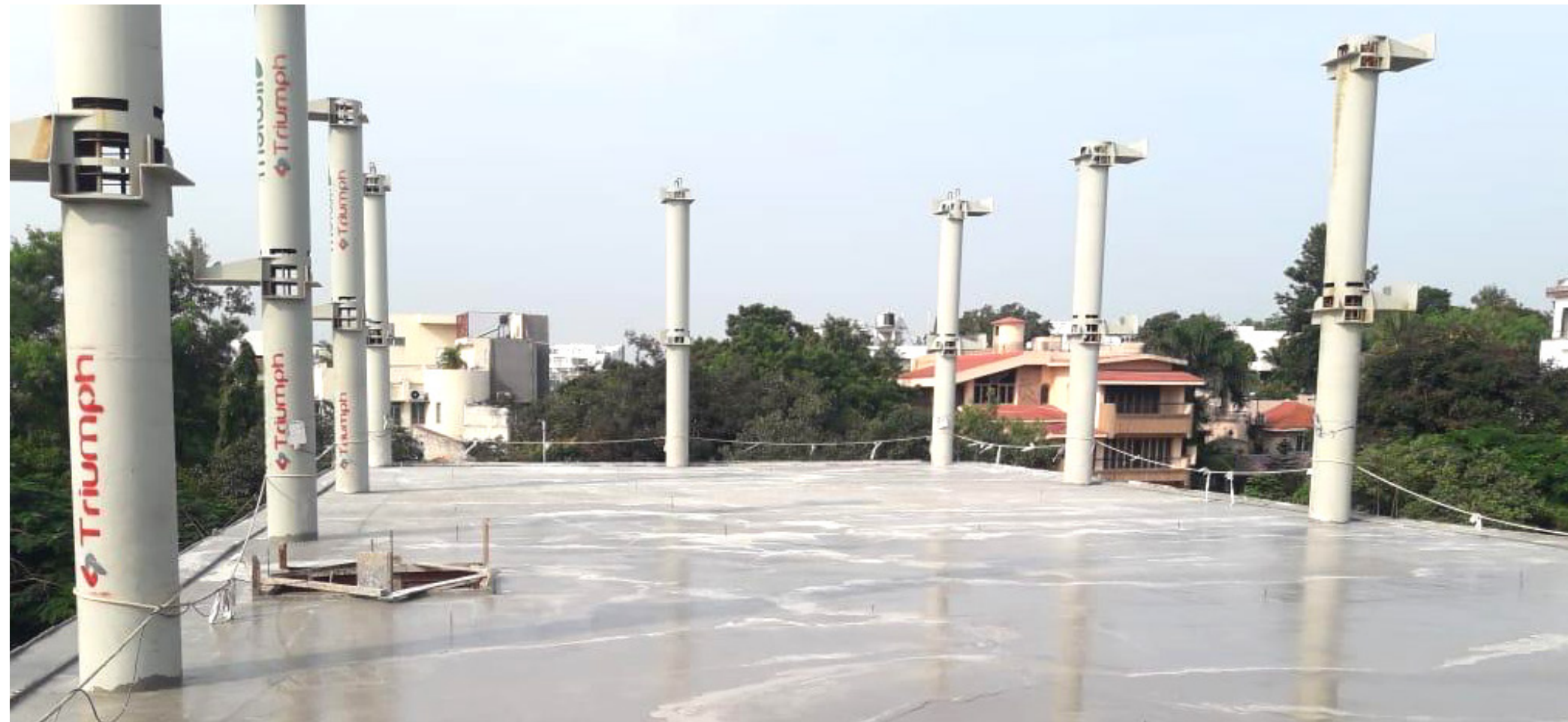
Multi-level REP columns with screeding
