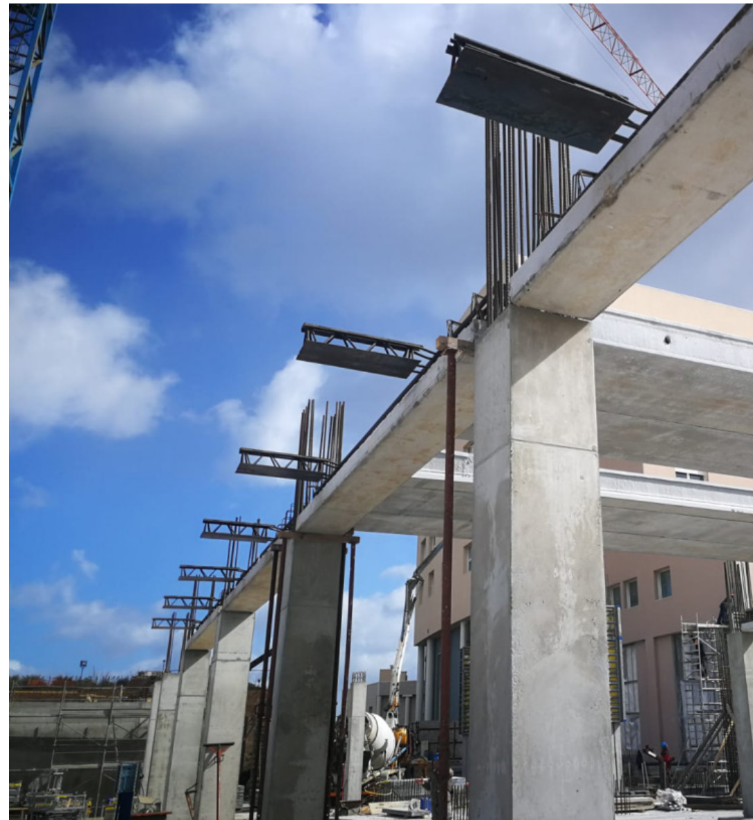
REP Cantilever Beams
