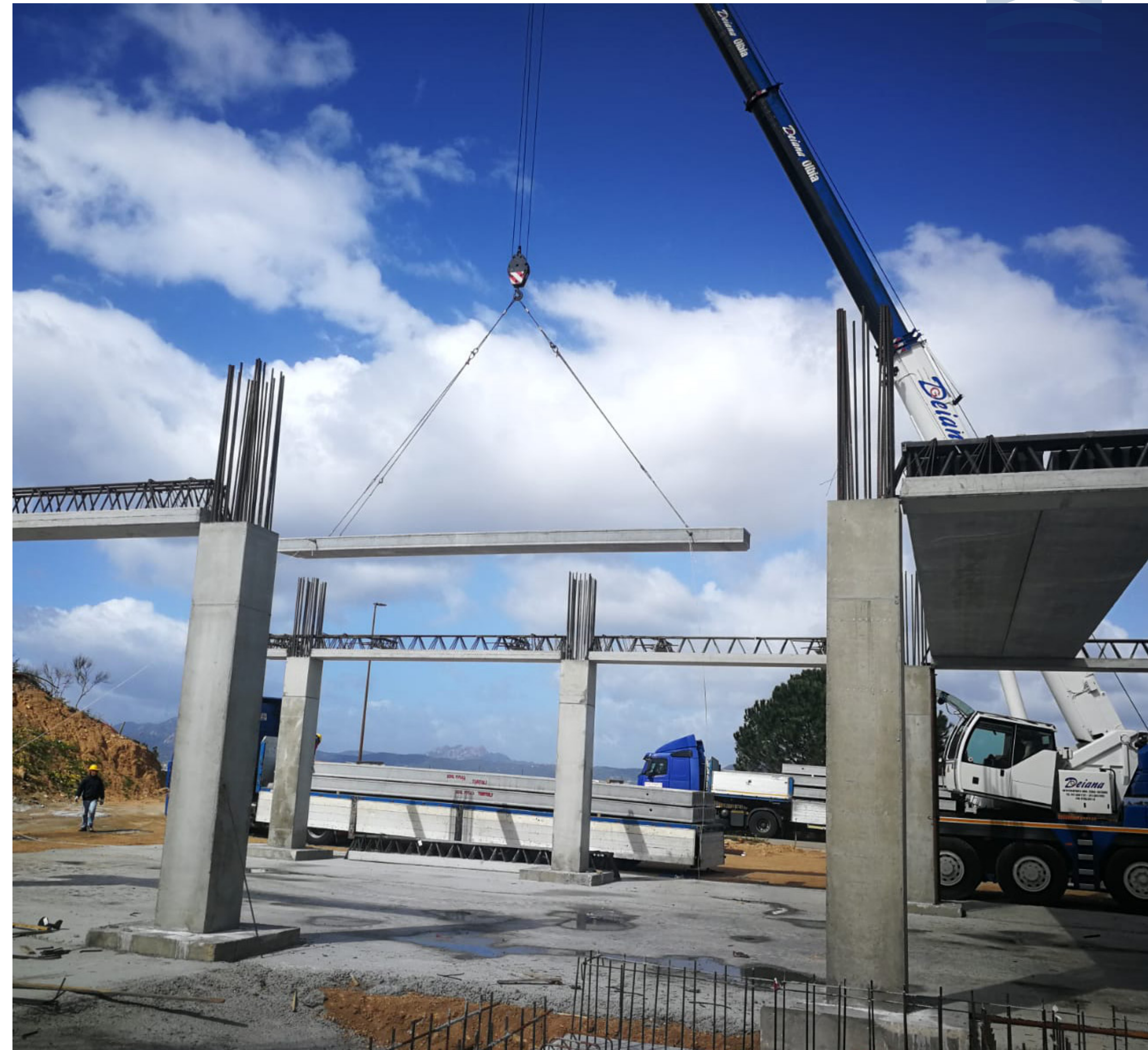
REP Beam on Precast Columns
