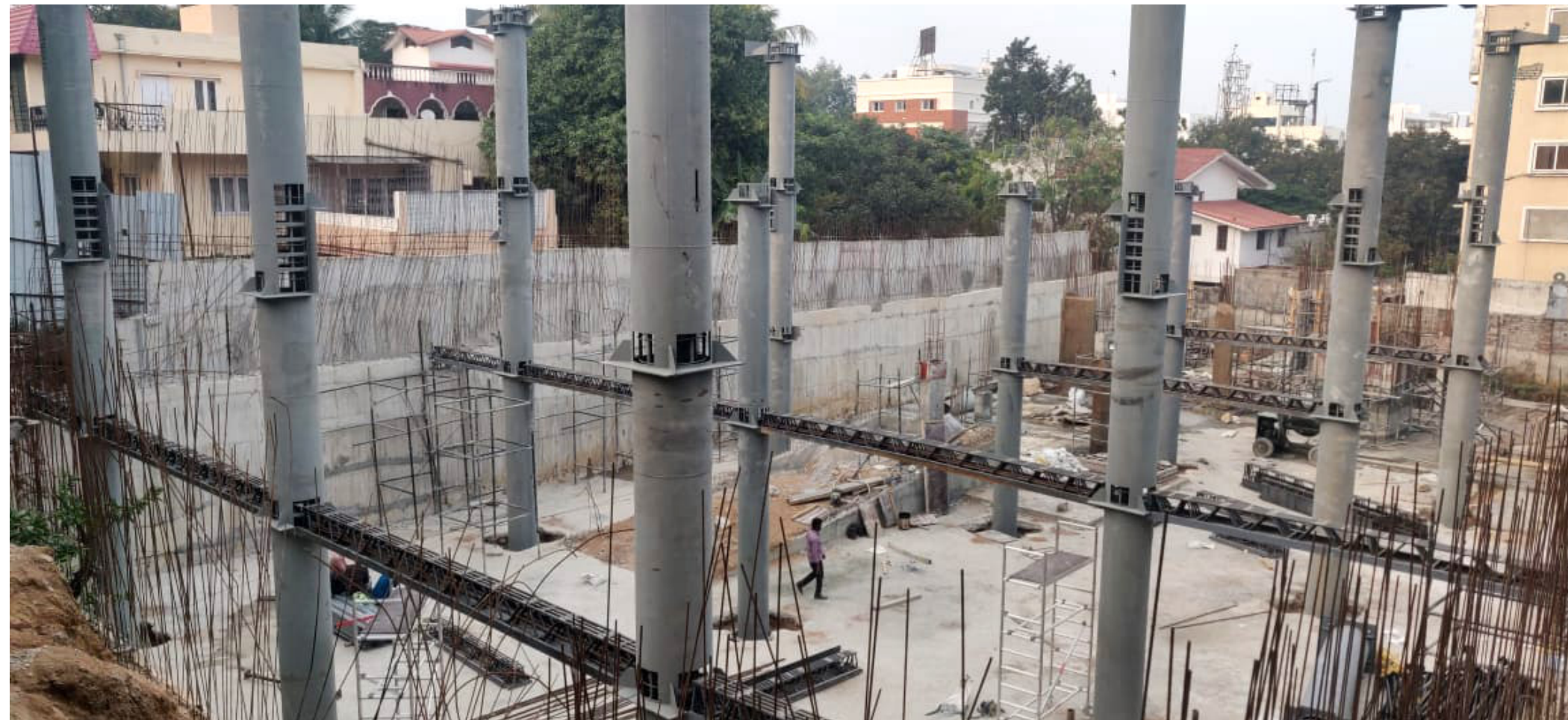
REP Beam & Column Framing
