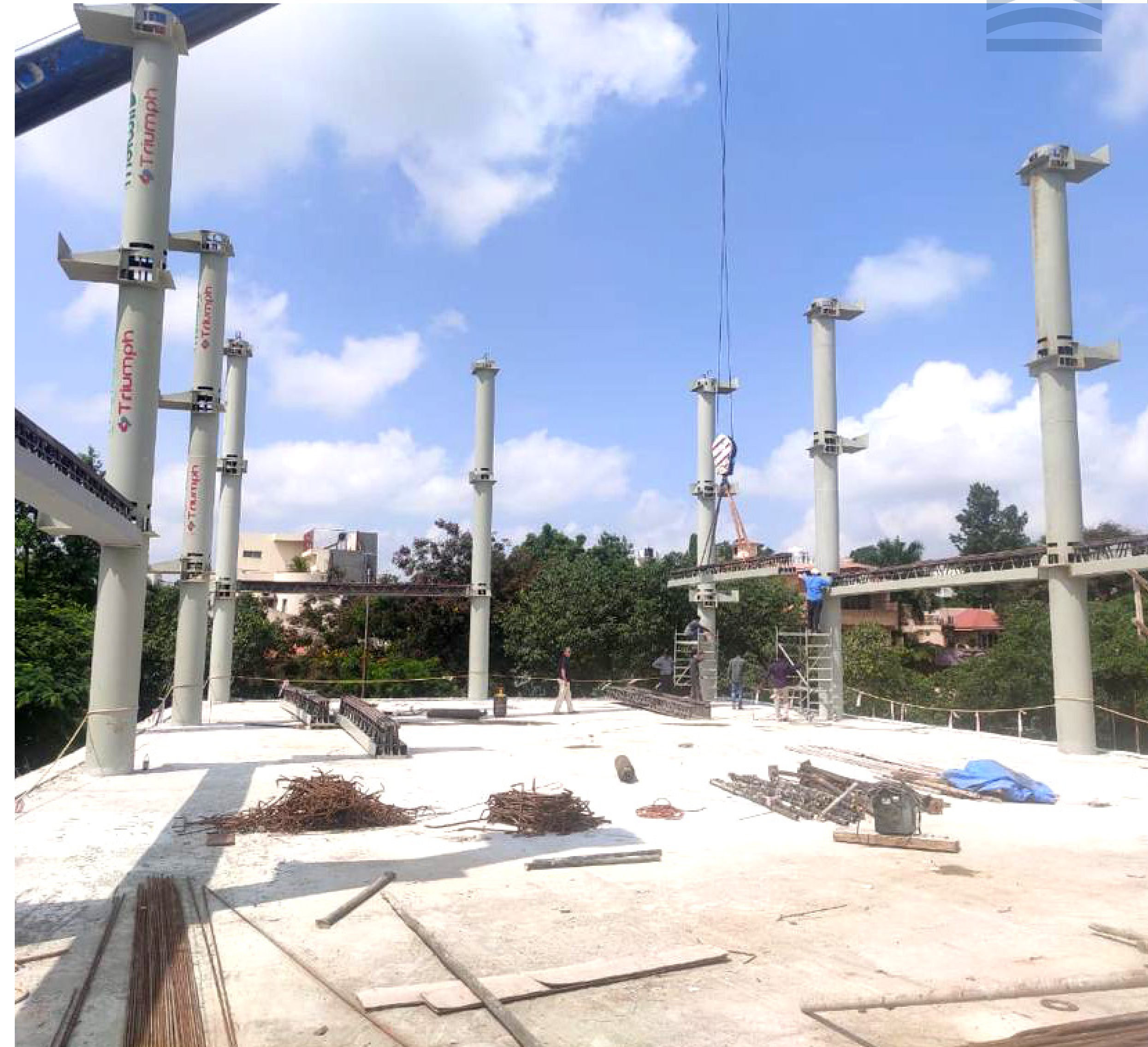
Multi-level REP columns
