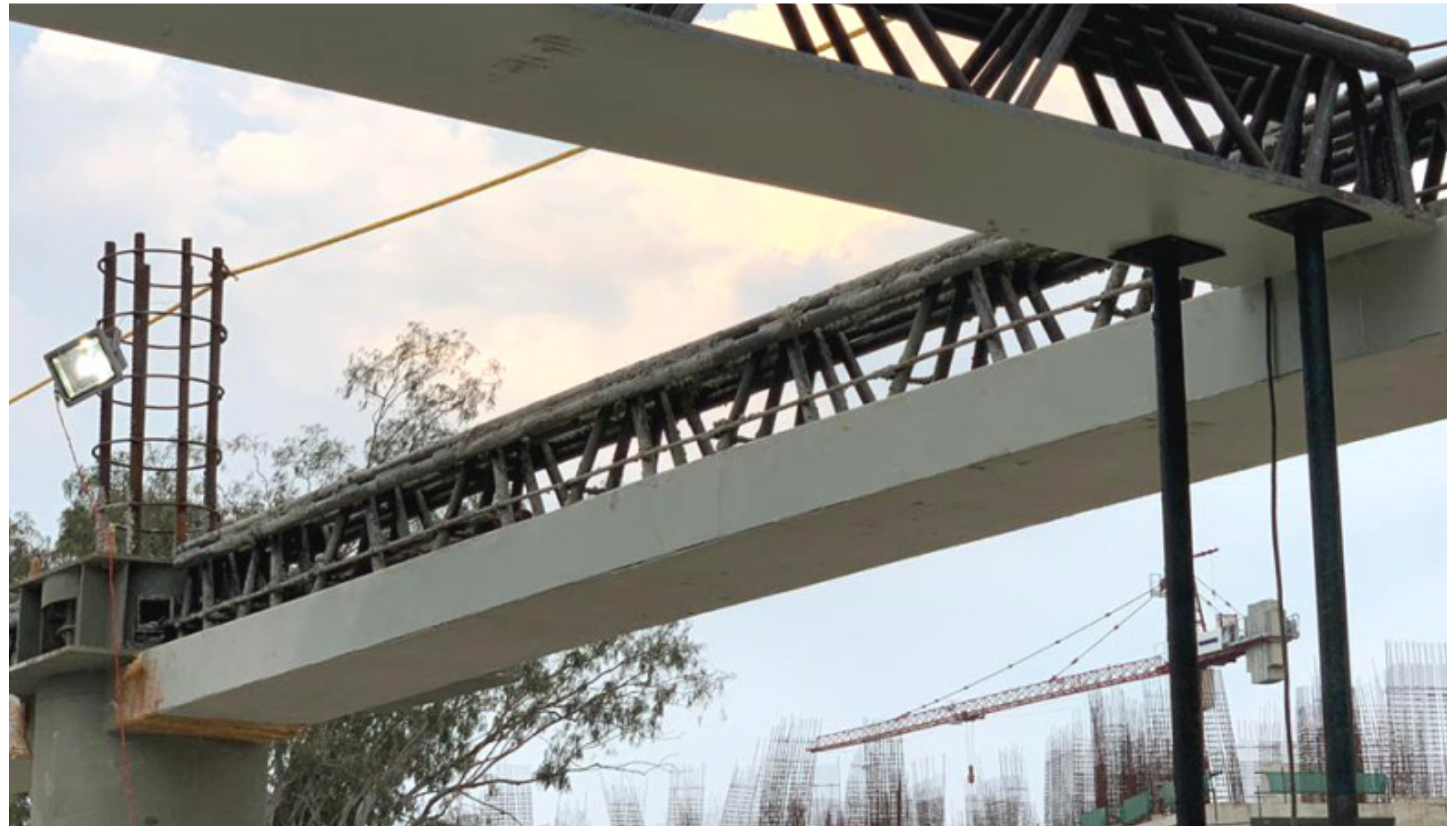
REP Beam to Beam connection
